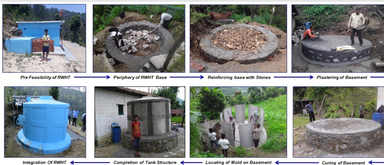
Figure 46: Sequence of building rainwater harvesting tank | Source: CHIRAG
