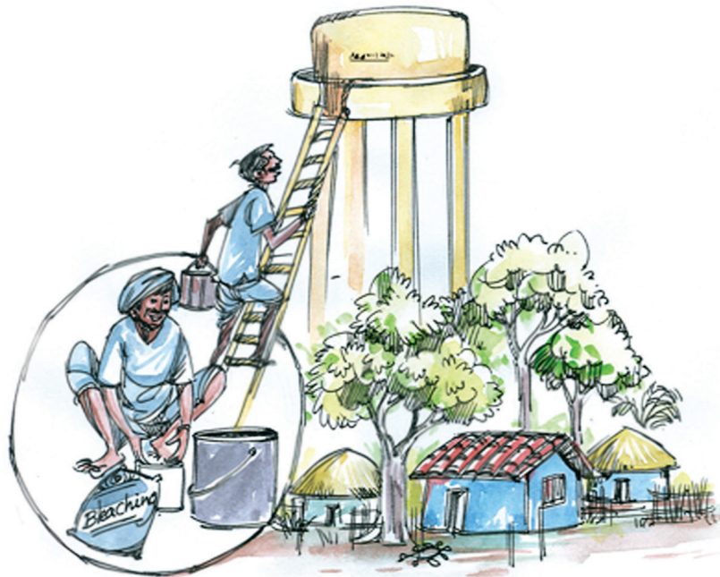
Chlorination of water in an overhead reservoir
