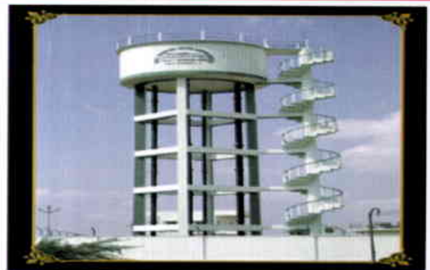
Over Head Balancing Reservoir (OHBR)
