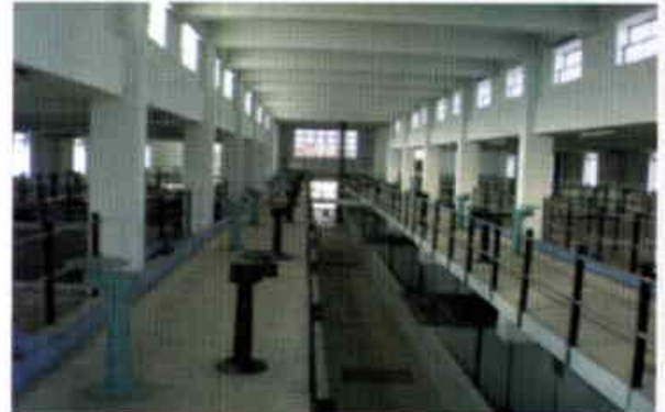
Filter Beds 16 filter beds, 5 x 6 m each size Design Flow : 2715 Cum/hr
