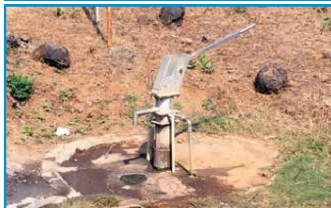
Solar dual pump installed in Maharashtra
