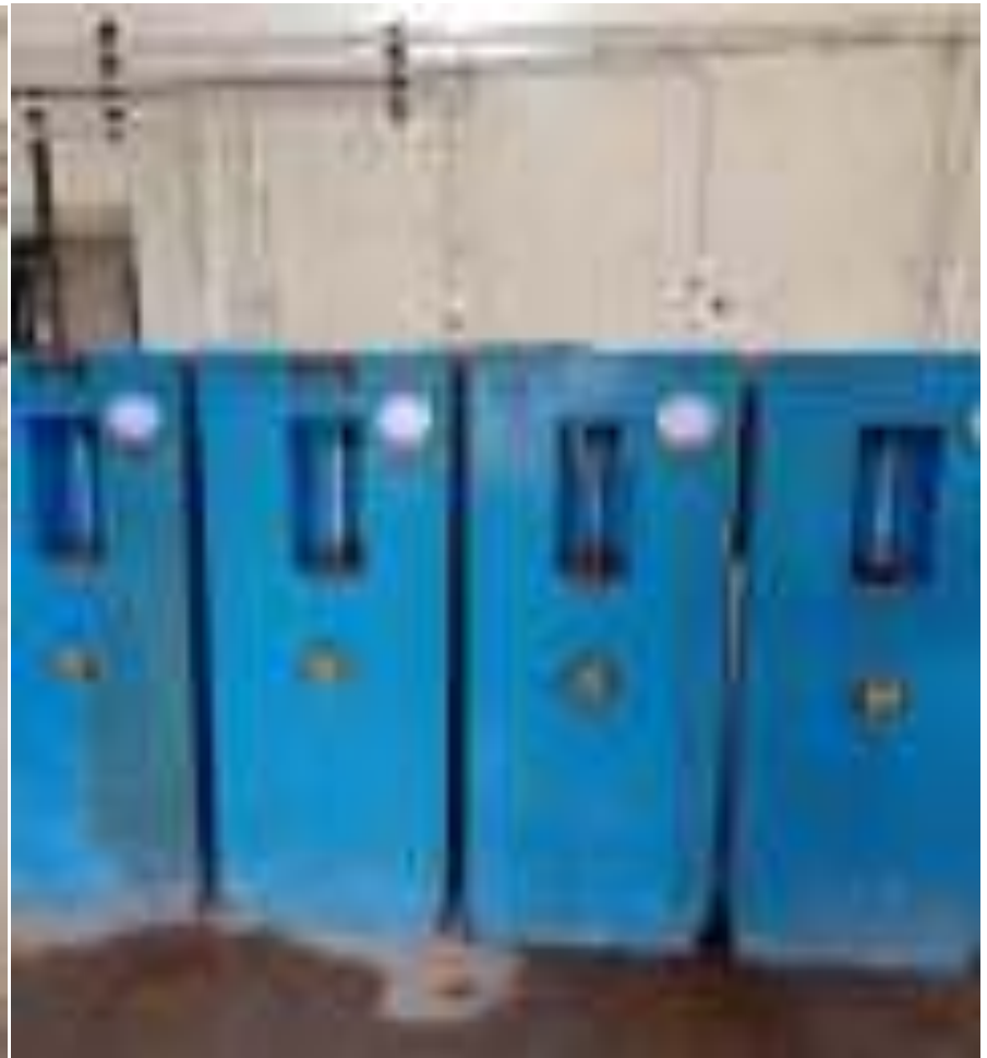
Chlorination of clear water through chlorine gas at Rukka water treatment plant
