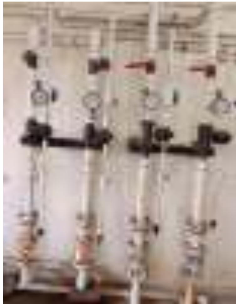
Chlorination of clear water through chlorine gas at Rukka water treatment plant
