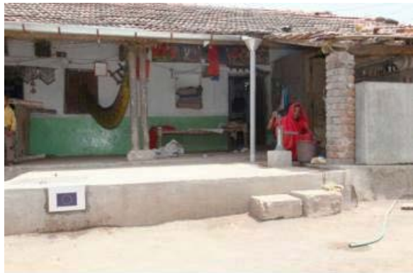
RRWHS at Kamlapur village, Surendranagar
