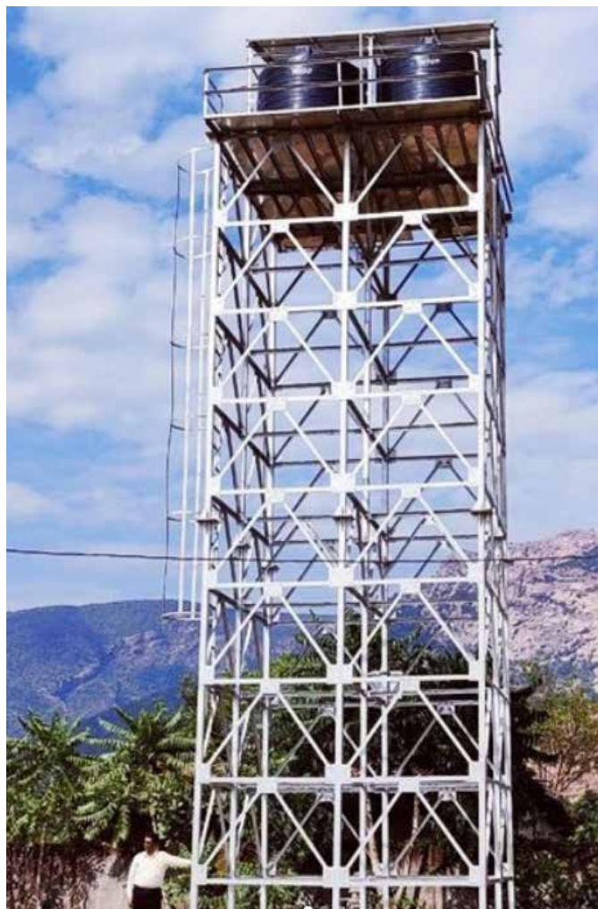
Figure 2 Solar-based system in Chhattisgarh
